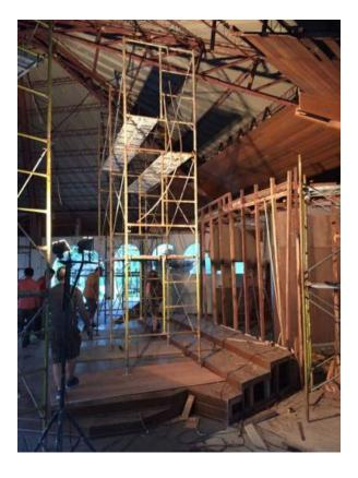
Some members of our team were working atop 30 feet of scaffolding under extreme conditions, with temperatures in the 30 to 32 degrees Celsius range. We found layers of supports under the metal circular roof where wooden framing had been secured by metal spikes and welded to the metal girders. Our top workers had to hammer these spikes loose after lowering the roofing boards to the floor. The best boards were saved and stored away for future use.
